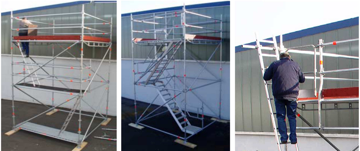
Fig. 5. Examples of installed access means
