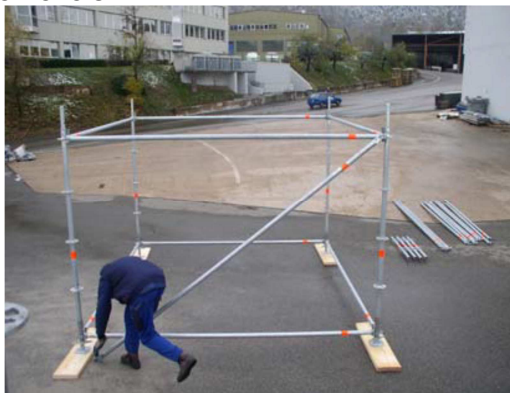
Fig. 4. Assembly of the first horizontal frame
