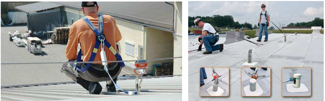
Fig. 2. Examples of horizontal safety systems
