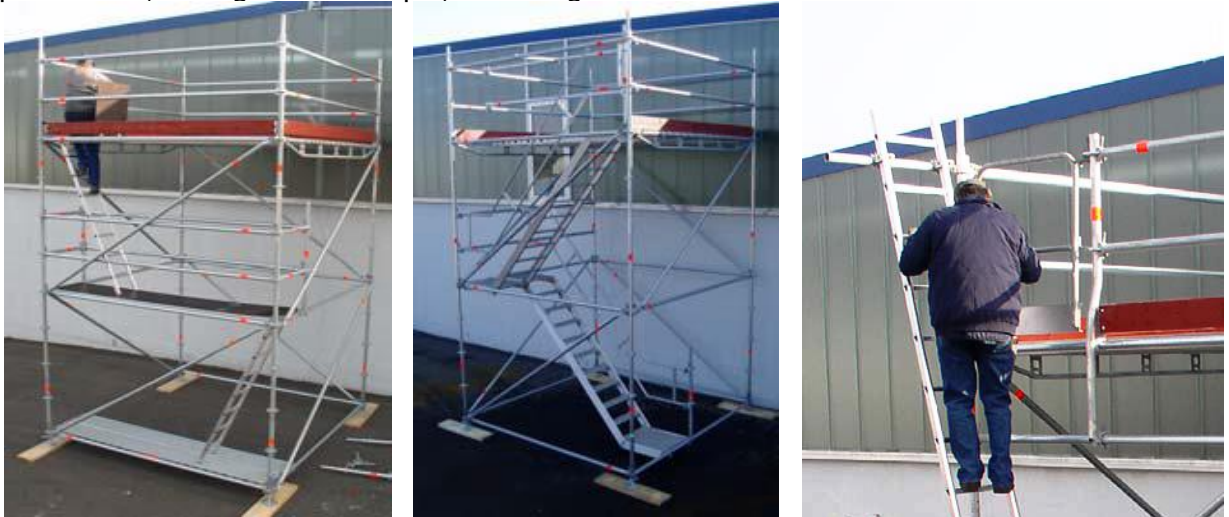
Fig. 5. Examples of installed access means
