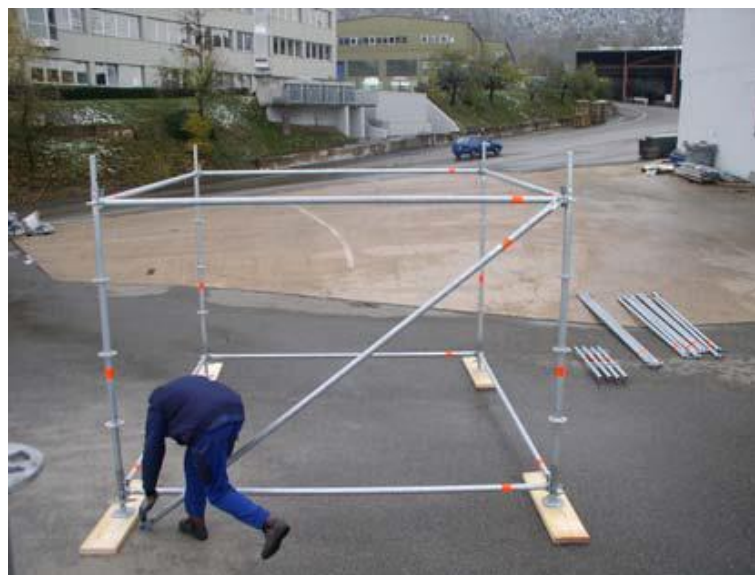
Fig. 4. Assembly of the first horizontal frame
