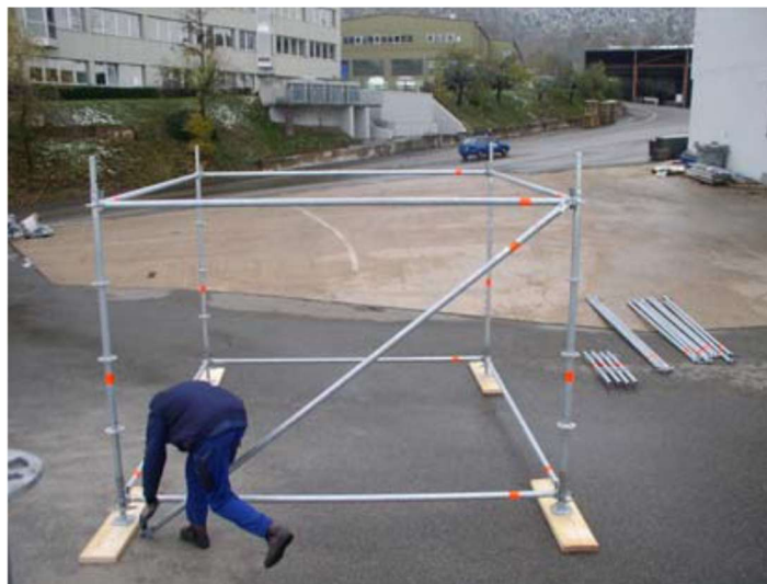
Fig. 4. Assembly of the first horizontal frame
