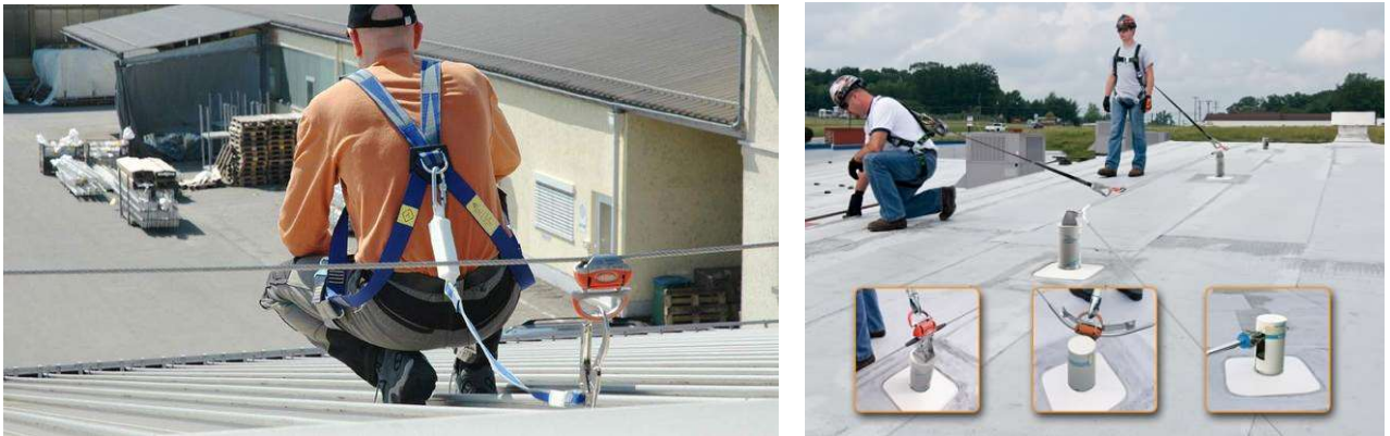
Fig. 2. Examples of horizontal safety systems
