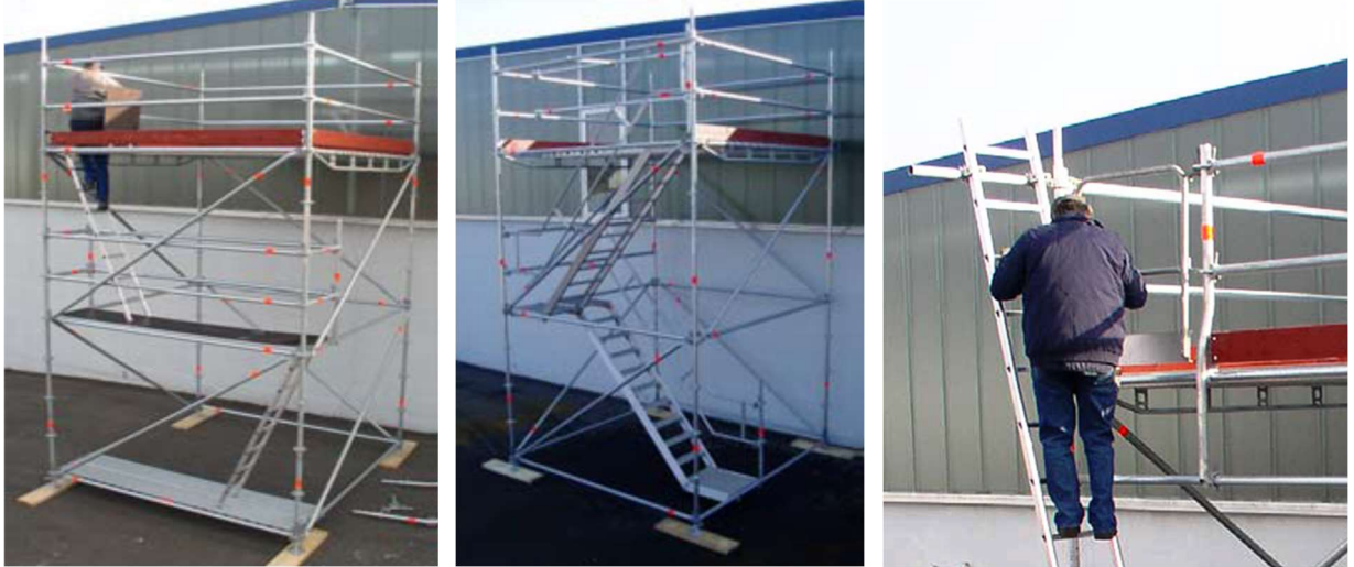
Fig. 5. Examples of installed access means
