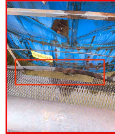
Repair of an opening in grating
