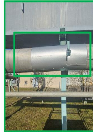
Repair of pipeline insulation
