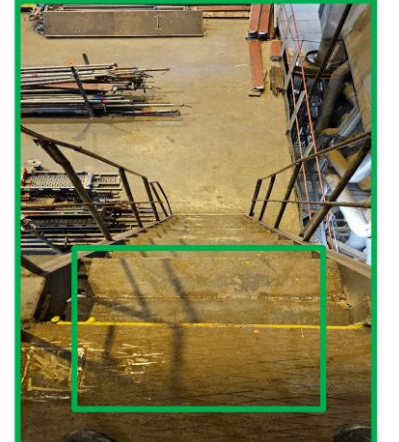
Unsafe manhole fixed and marked
