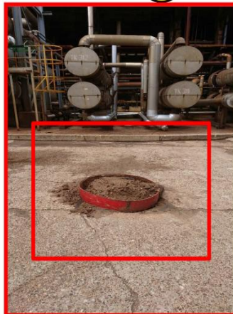
Repair of an unsafe sewer well
