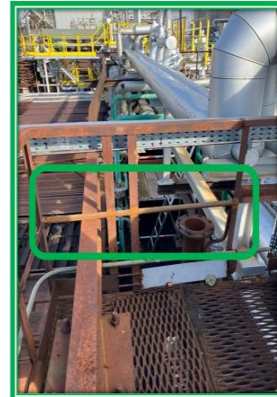
Installation of a safety guardrail
