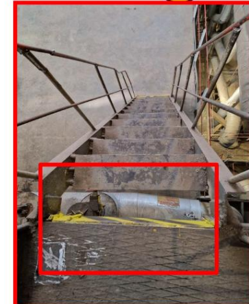
Unsafe manhole fixed and marked
