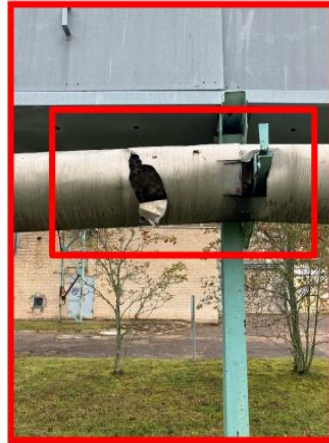
Repair of pipeline insulation
